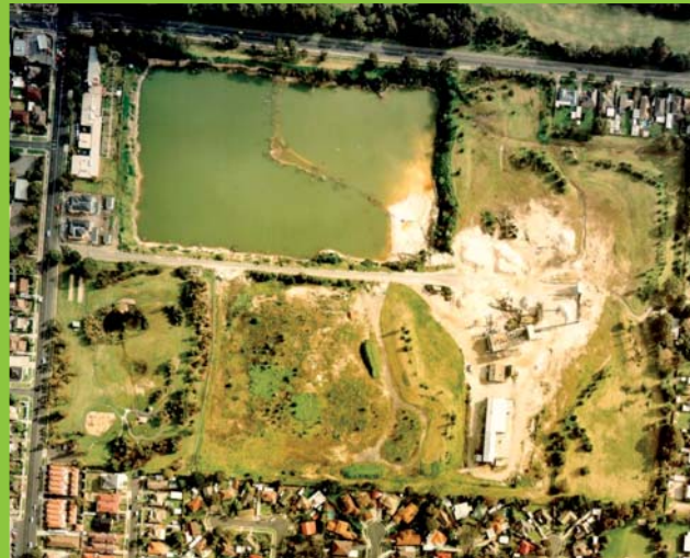
An aerial view of the quarry redevelopment site in Huntingdale with the adjoining golf course that the water will be supplied to.
